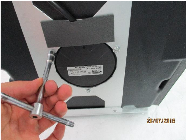
7. Unscrew the condenser's fan (3 bolts) and remove it
