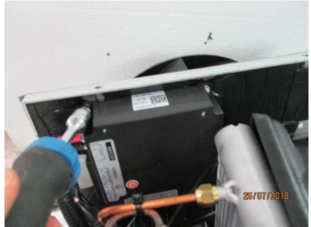
8. Unscrew the 2 upper bolts of the ECU and rotate it
