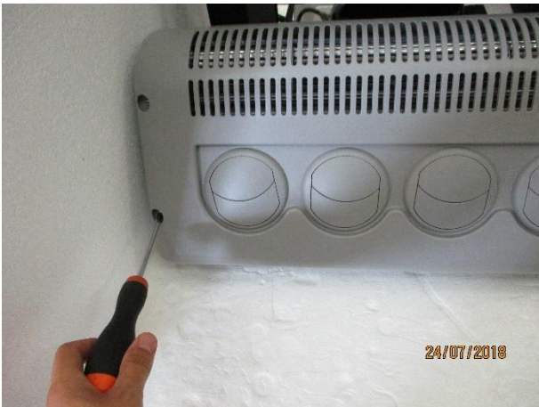
1. Unscrew the air diffuser (4 bolts)
