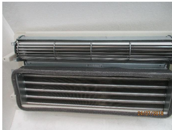
3. Remove the evaporator blower and reverse the procedure to replace it
