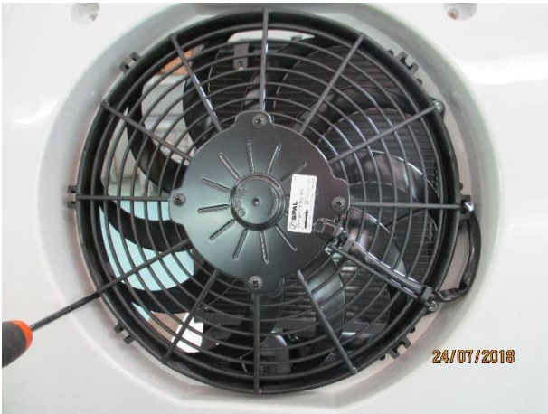
1. Unscrew the condenser fan (4 bolts)
