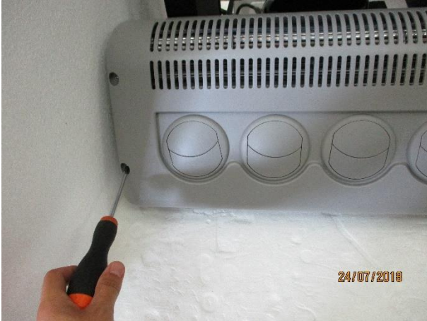
1. Unscrew the air diffuser (4 bolts)
