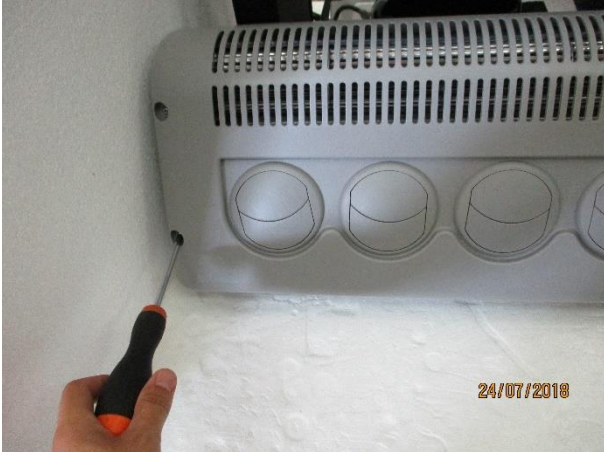
1. Unscrew the air diffuser (4 bolts)
