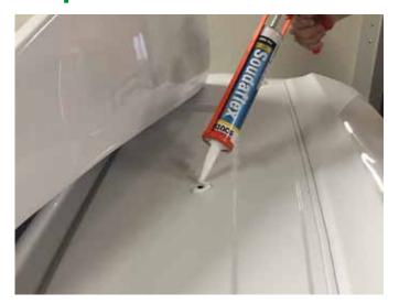
Run a generous bead of sealant around both holes to help create a water tight seal.
