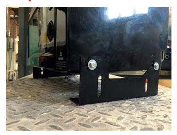
Secure legs as shown to either side of the microwave unit. Use supplied short bolts and washers.
