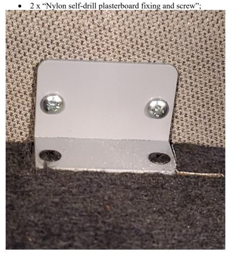
Step 6: Fit the "Fibreglass locker fascia" into the "Scania top bracket 0636" using:
