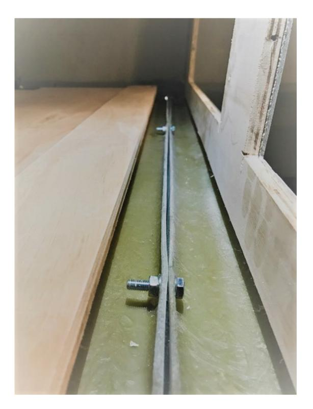
Fix facia to locker floor, as shown above. Secure using M6 x 25mm Screws, M6 x 12mm Washers & M6 Nyloc Nuts. Tighten all fixings.
