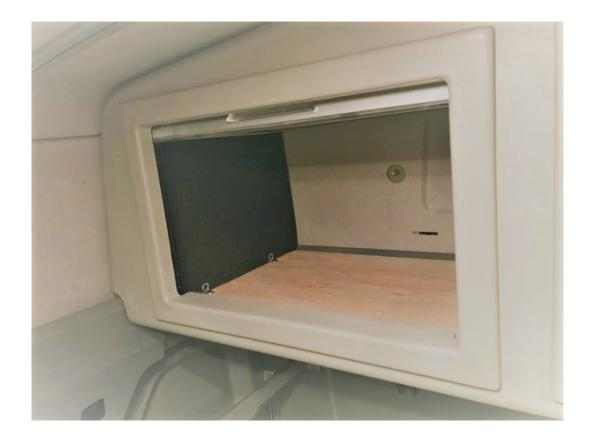
Fit 3 x door surrounds onto front, locating bonded in screws through pre drilled holes in facia.
